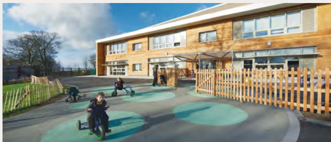
↑ Bushbury Hill Primary School near Birmingham is another of Architype’s UK Passive House schools. Image: Architype/ Leigh Simpson Photographer
