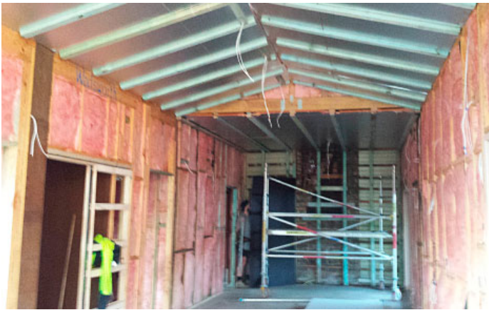
↑ Insulation installation in walls and ceiling.
