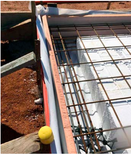
↑ Waffle pod slab before (left) and just after the concrete pour. Note the termite barrier under the waffle pods, as per the ISEG.2 approach.
