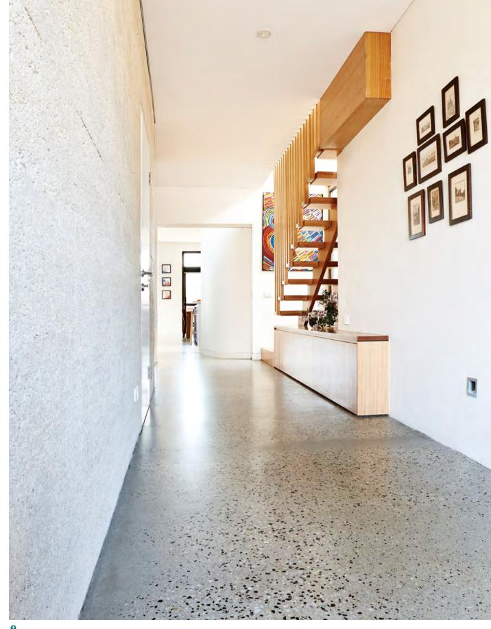
This Melbourne home's polished concrete floor includes 30 per cent flyash with a lovely aggregate pattern exposed in polishing. The slab edge is insulated with R1.5 Foilboard and the floor is finished with Kunos Natural Oil by Livos. Image: Rhiannon Slatter. There is a profile of this Steffen Welsch Architects design in *Sanctuary* issue 25.
