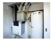
The mechanical ventilation system with heat recovery (MVHR) for a single-family home is typically only the size of a clothes dryer and is often installed in a cupboard in the laundry or hallway. The ducting is concealed in the ceiling with small vents in each room. The system is very quiet and uses less energy than a 50w halogen light bulb.
