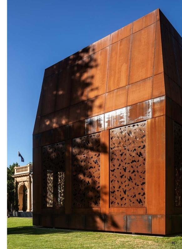
Maintaining a AA-standard environment for both the gallery and storage spaces could have made for expensive running costs. However the chosen combination of high levels of insulation, an airtight envelope and an energy recovery ventilation system have produced a highly energy-efficient building, slashing operational costs for mechanical systems and delivering a space that is very comfortable to occupy.
